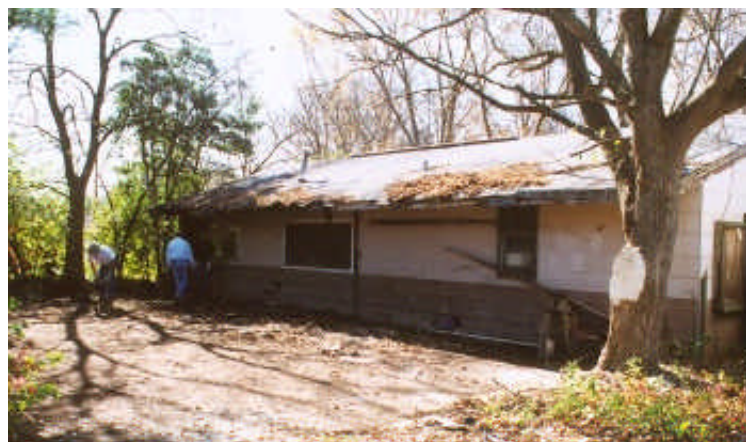
Look, there was a concrete pad under all those weeds.
